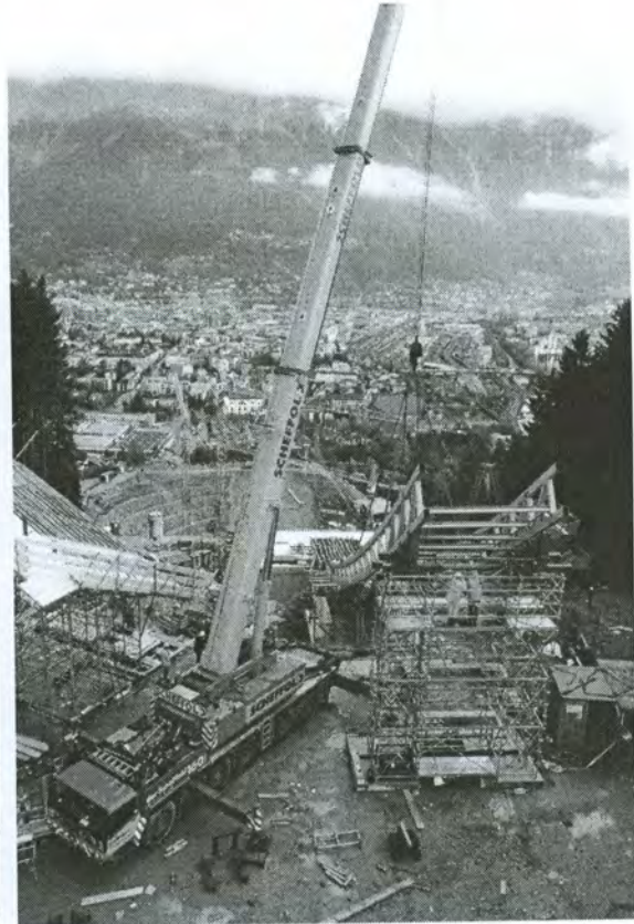
Fig. 10 - Lifting of the first part of the approach ramp
