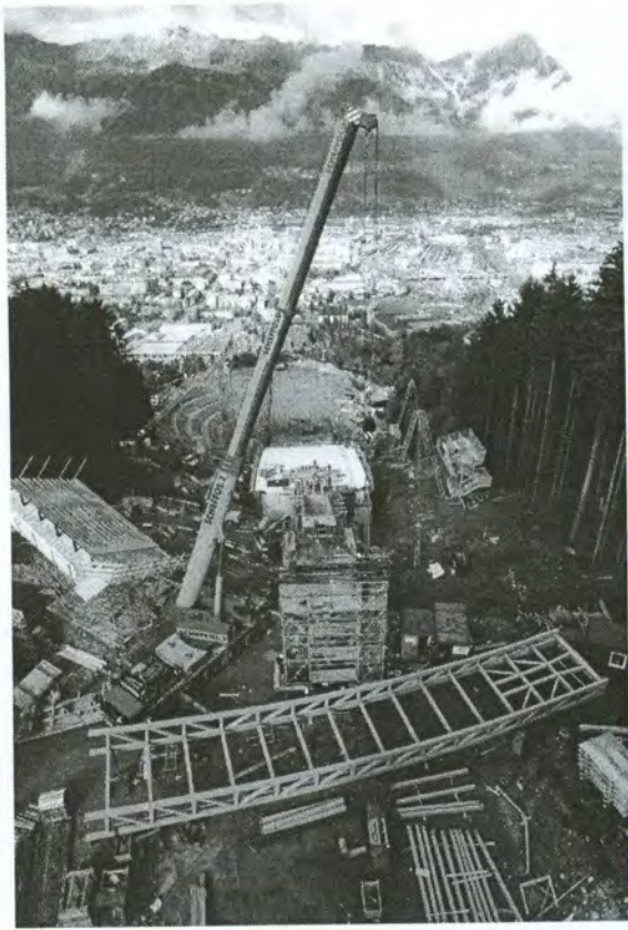
Fig. 10 - Lifting of the first part of the approach ramp
