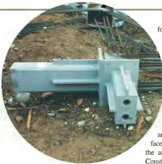
Figure 6: LEFT AND ABOVE – The docking station between the concrete tower and steel cage with prestressed bearing plates.
