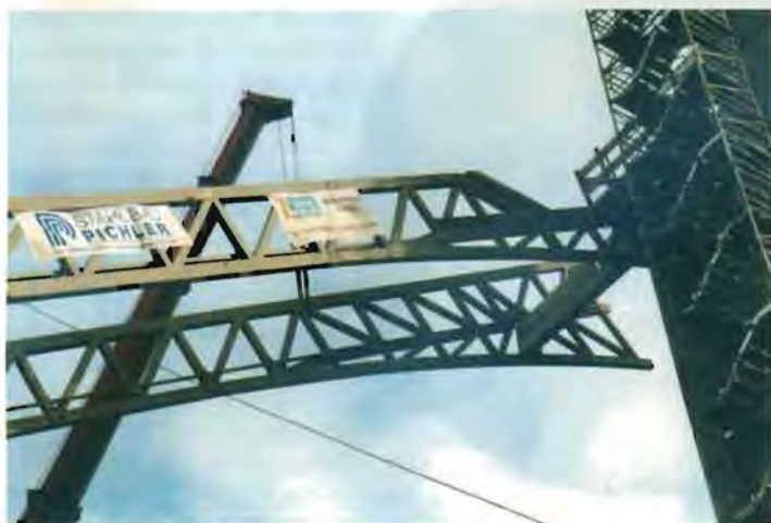
ABOVE: Figure 3: Lifting the second part of the approach ramp.
