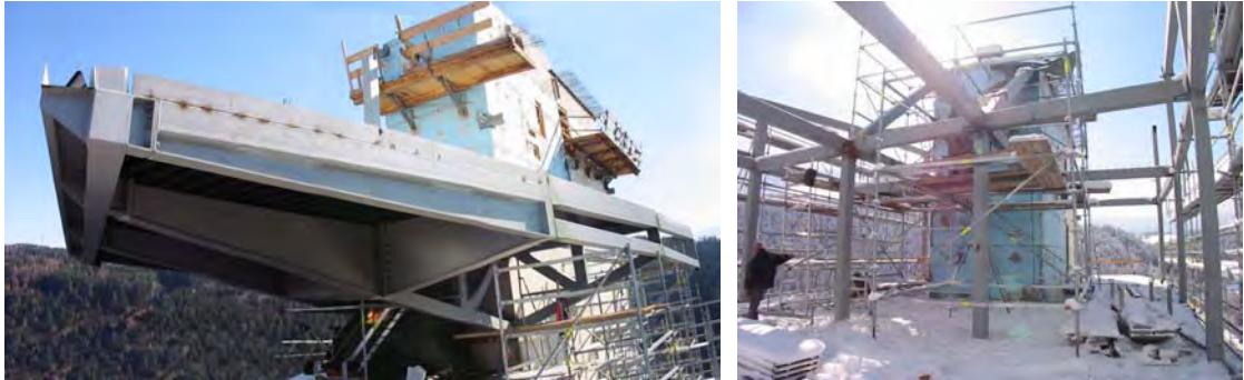
Figure 6. Cantilevering steel cage during construction.
