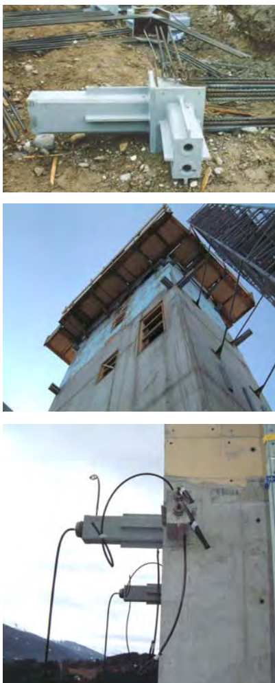
Figure 7. Pre-stressed docking devices.
