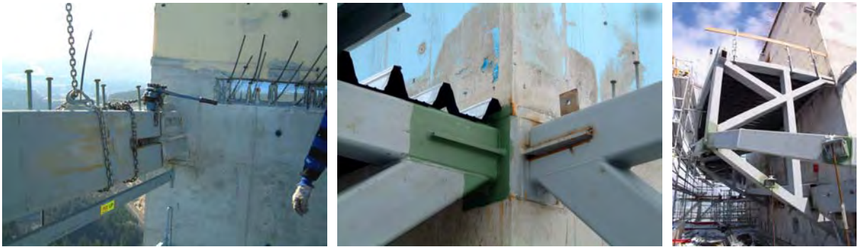
Figure 5. Slotted hollow sections welded to the docking brackets.
