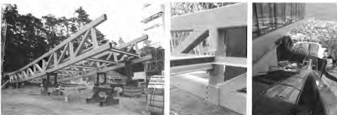
Fig. 9 Approach ramp - steel truss trough bridge
