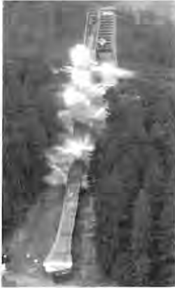
Fig. 2 Blasting of the old olympic ski jump
