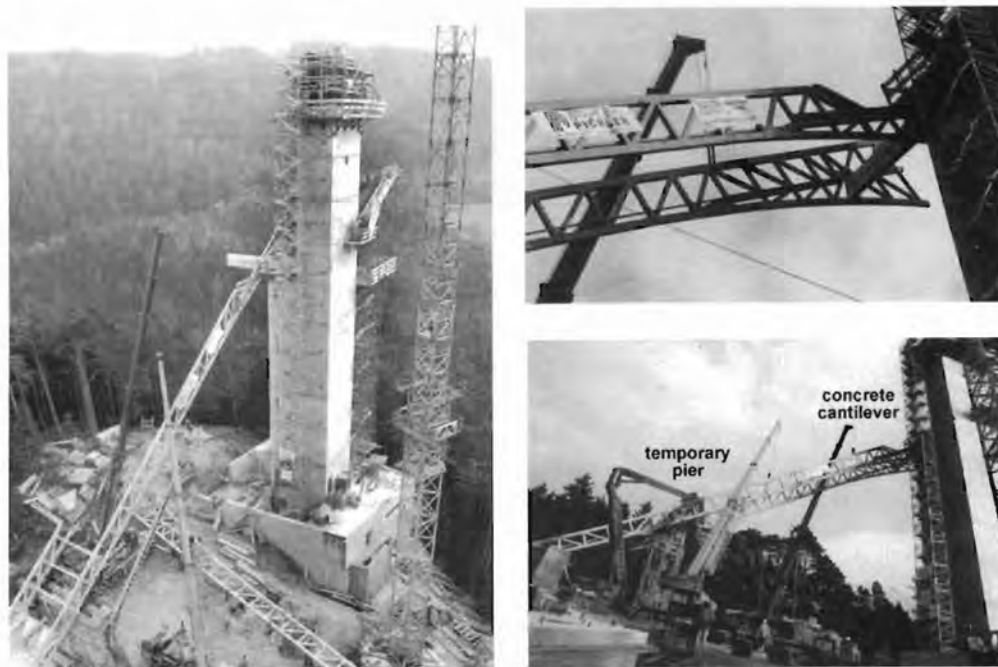
Fig. 11 Lifting of the second part of the approach ramp
